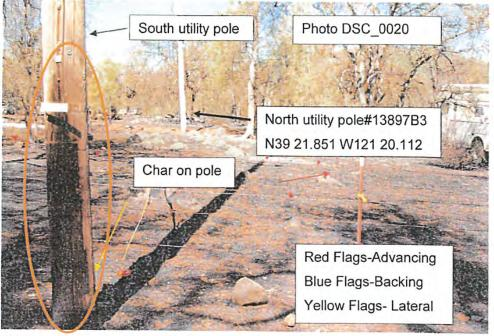
Examining the lines from the bucket truck I observed the AT&T communication lines had sooting on them. I could not visually see any damage to the AT&T communication lines attached between the two poles.
